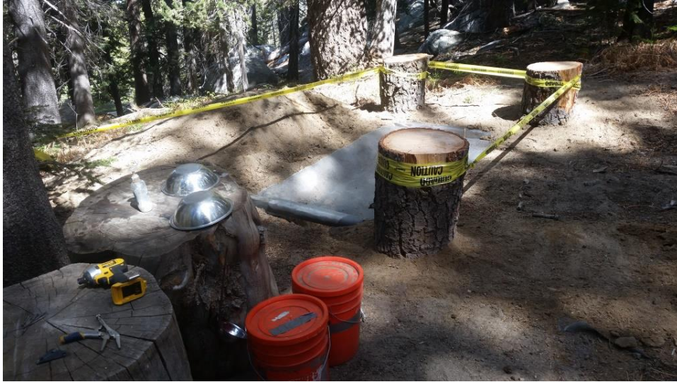
Photo 19.4 - Grey Water Sump
